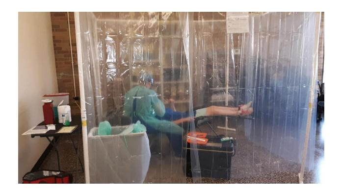
Michigan has a program using a "school operatory" designed by a dental hygienist and her engineer neighbor. The space was created using PVC pipe and shower curtains. The PVC pipes come apart and are easily transportable in a bag.
